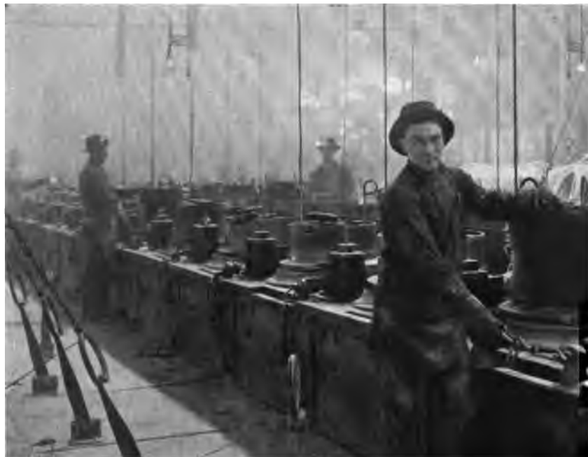
Fig. 1. Automatic Stops for Drawing Blocks.*
